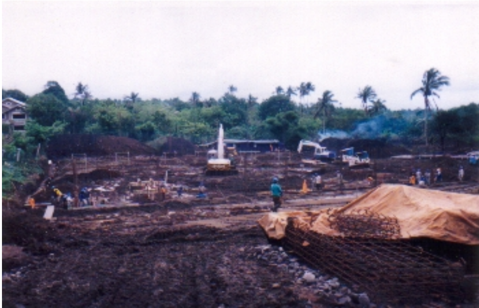
PGA Geopier crew on the job at CBCP-NASSA Training Center
