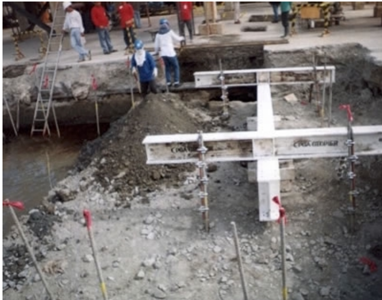
Modulus Load Test Setup
