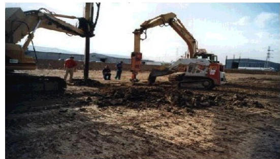
Fig. 1.4 Typical GEOPIER Construction Equipment consisting of Auger, Tamper and Feed Loader.
