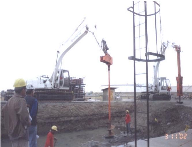
**Picture 1 - Auger Machine for excavation of hole**
