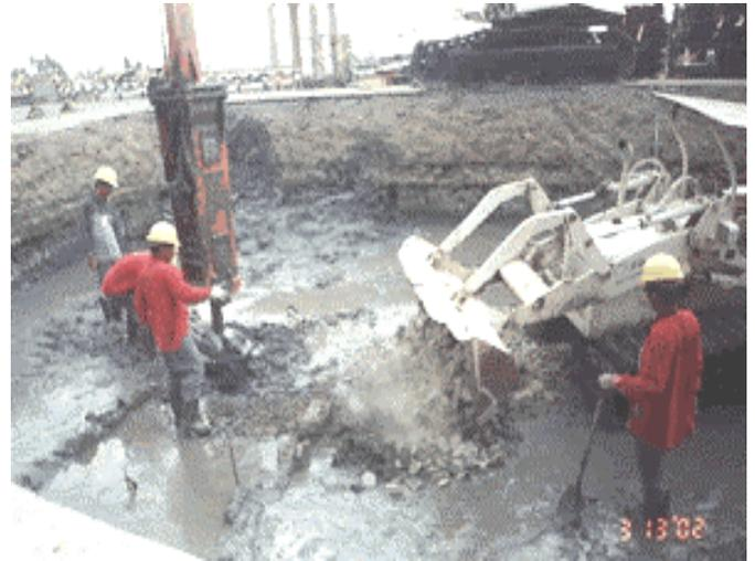
**Picture 2 - Aggregate being lowered into hole in increments**
