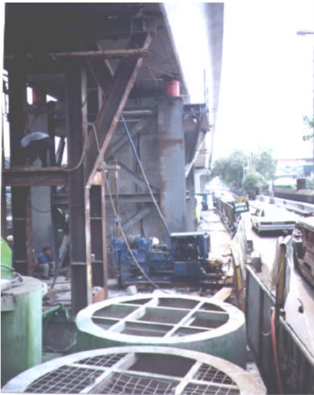
Fig. 6 – Jet Grouting Equipment Layout
