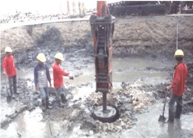
**Picture 3 - Hydraulic Hammer with Bevelled Rammer being lowered into the hole**
