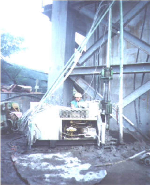
Fig. 5 – Jet Grouting Machine set up under Pier
