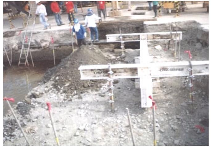
**Picture 4 - Geopier Modulus Load Test Setup**
