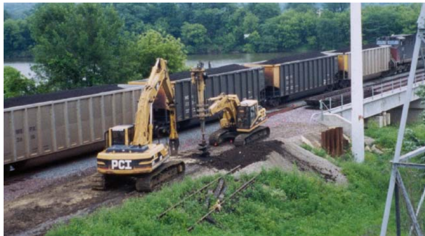
Fig 4.2 - Conventional GEOPIER Installation Equipment
