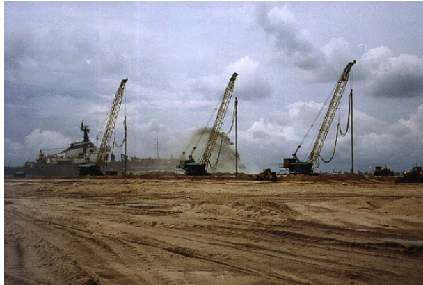
Figure Picture Showing Vibroflotation Equipment
