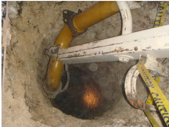
Fig Sealing of the tunnel using pumpcrete and highly flowable concrete
