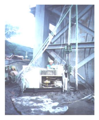
Fig. 6. Jet Grouting Machine set up under Pier
