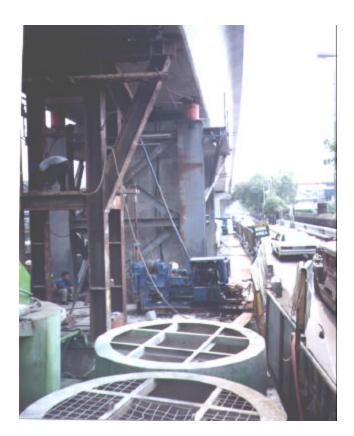
Fig. 7. Jet Grouting Equipment Layout
